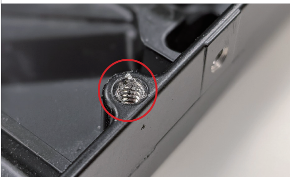
Damaged screw hole
